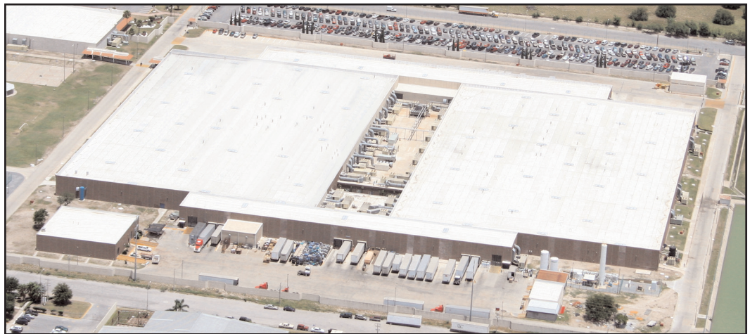
The Delphi Reynosa is just one of the large, Carlisle projects completed by CUBIMSA's in 2006. For the past two years, CUBIMSA has been Mexico's largest installer of Carlisle single-ply systems.
